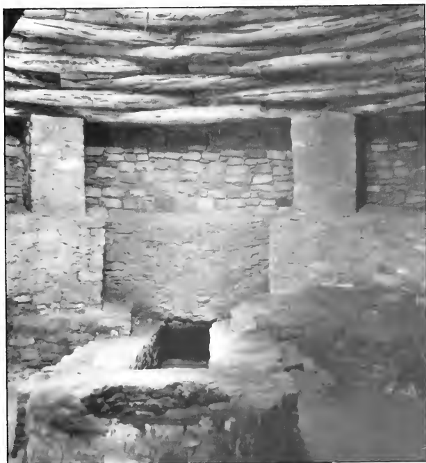
Figure 3.12. Interior of Kiva E, showing reconstructed cribbed-log roof.
